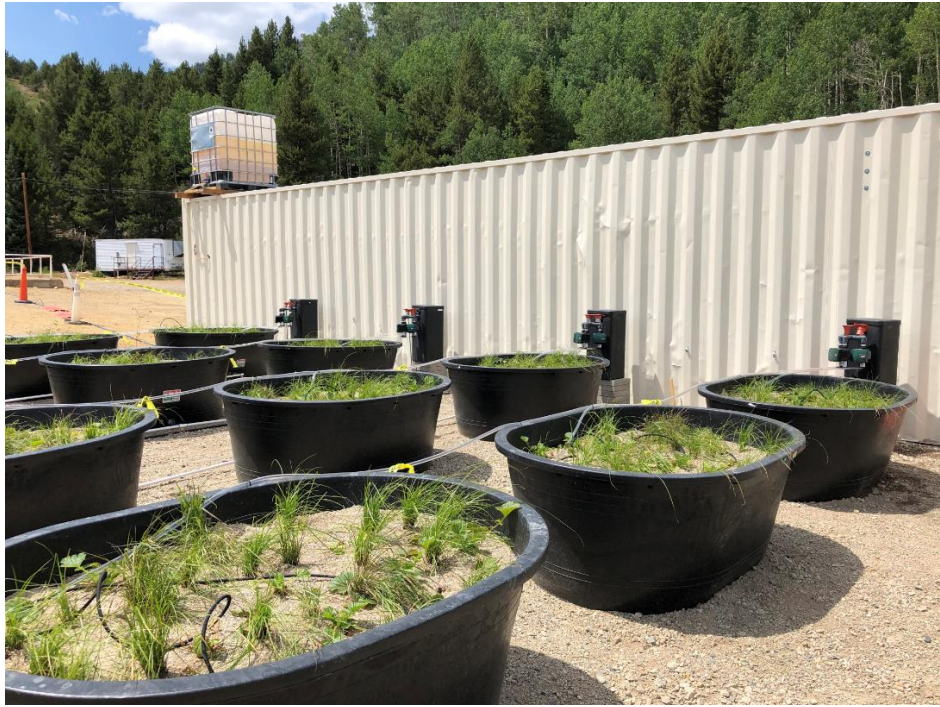
Figure 5: Vertical flow wetland as the final treatment stage
